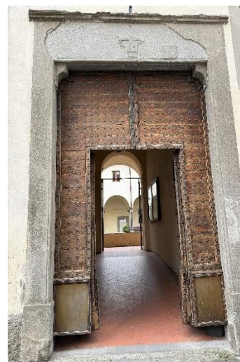
8 secondary entrance on the floor
